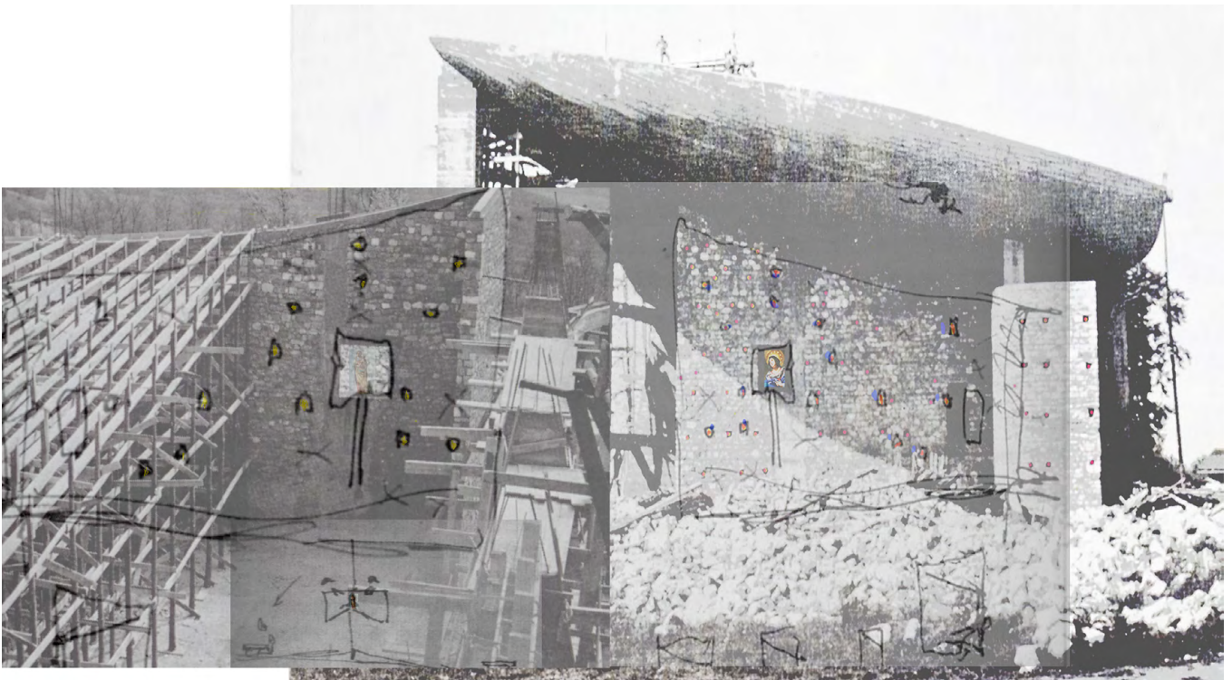
Figure 5. Montage: "Look! Here are your stars!" Construction photos with Le Corbusier's sketches overlaid the grid of scaffolding holes. © Marcia F Feuerstein 2019.
